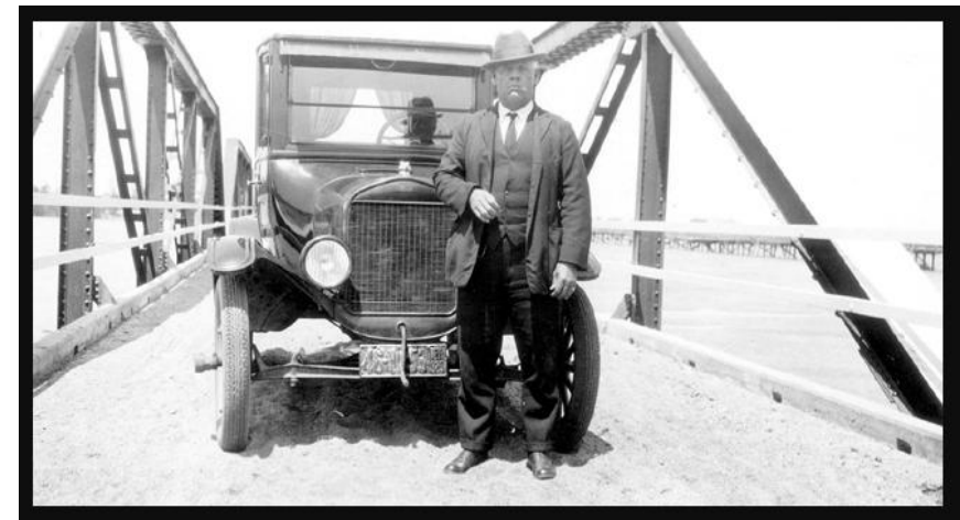
Wahoo, NE – First car over the Silver Creek Bridge in 1925 Courtesy of Nebraska Department of Roads
