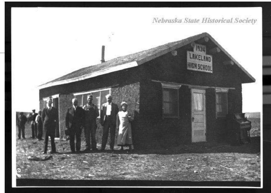
Johnstown, NE – Lakeland sod high school completion in 1934 Courtesy of Nebraska State Historical Society
